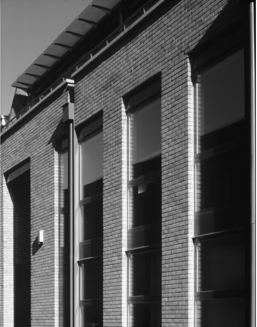
Figure 1.2 Simon Foxell's projects rarely go beyond £1.5 million in value, for which he will charge a fee of 6-8 per cent.
