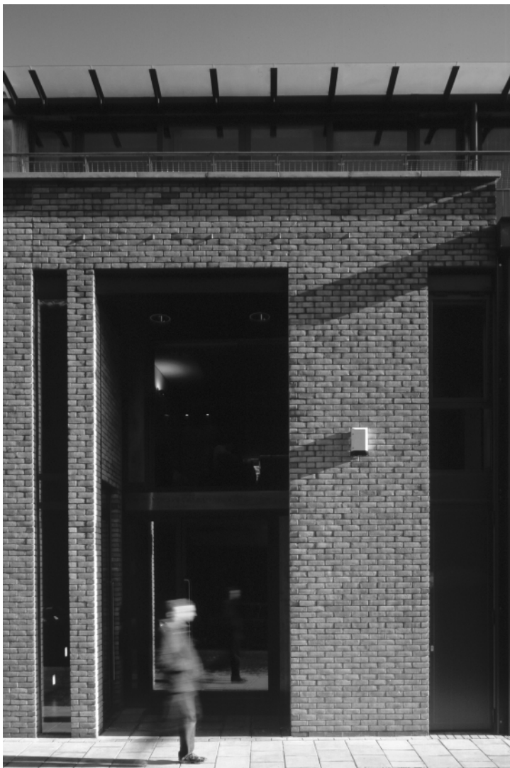
Figure 1.1 Boston Place, London, by Simon Foxell. A modern insertion in brick and expressed steel.
