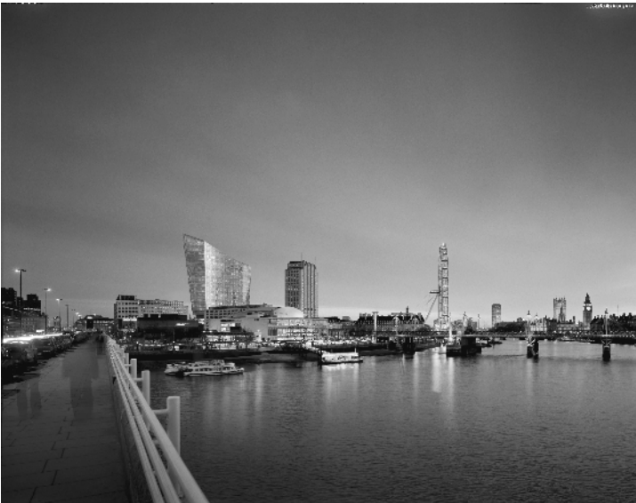
Figure 5.1 Controversial tower proposal from RHWL, for a site near Waterloo station, London.
